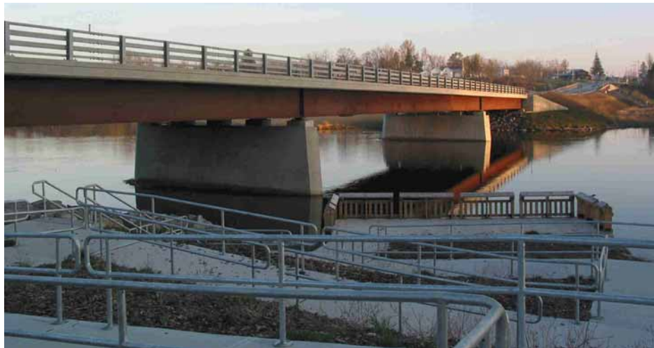
FIGURE 4 Completed Salmon River Bridges.
