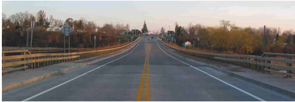
FIGURE 3 Salmon River Bridge (looking south).
