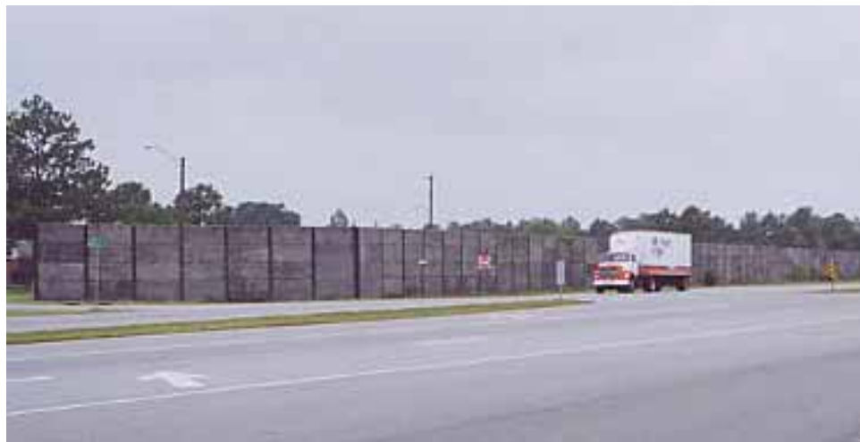
FIGURE 4 Noise walls in Section C.
