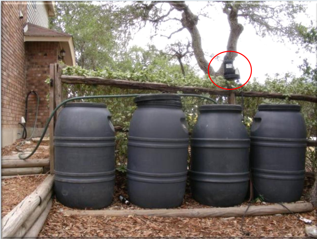
One-Third Horsepower Sump Pump Moves Water From Storage
