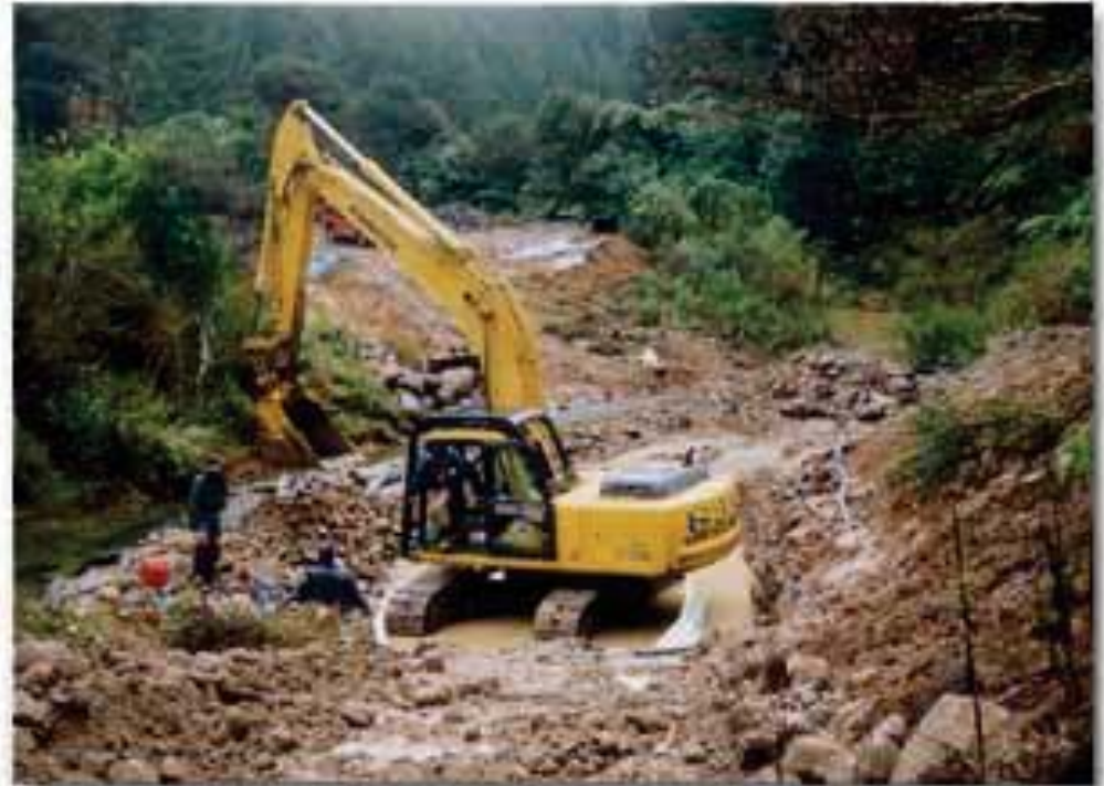
Stream crossing construction
