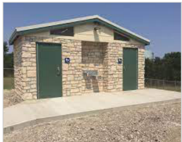
BATHROOM FACILITIES AT CROSS MOUNTAIN PARK IN FREDERICKSBURG BUILT USING PARKLAND DEDICATION FEES. IMAGE COURTESY OF THE CITY OF FREDERICKSBURG
