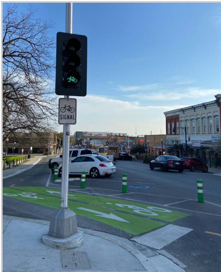
SIGNAGE, PAINTED BIKE LANES, AND CURB EXTENSIONS SUPPORT TRAFFIC CALMING IN DOWNTOWN SAN MARCOS. PHOTO COURTESY OF LEAH CUDDEBACK
