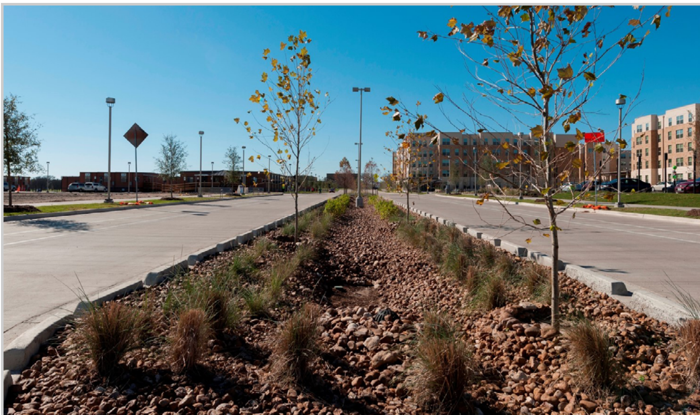
ROCK BIORETENTION ZONE IN A HOUSTON PARKING LOT. PHOTO COURTESY OF DAVID BATTS, CONSTRUCTION ECOSERVICES
