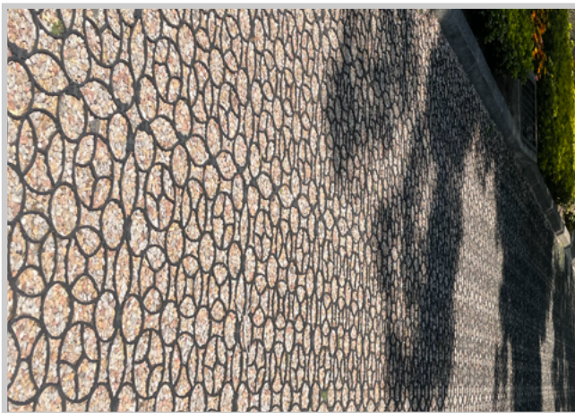
GRID PAVEMENT SYSTEM. PHOTO COURTESY OF MAGGIE NEMETZ
